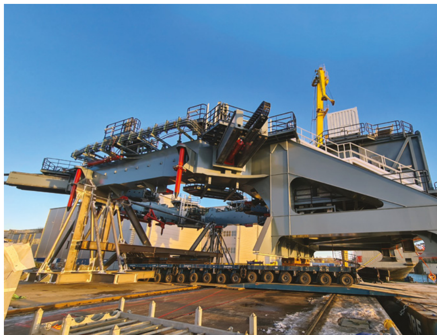
Motion-compensated gripper is transported onto a barge, in preparation for lifting on board Seaway Strashnov , in readiness for the first commercial monopile installation in DP mode.
